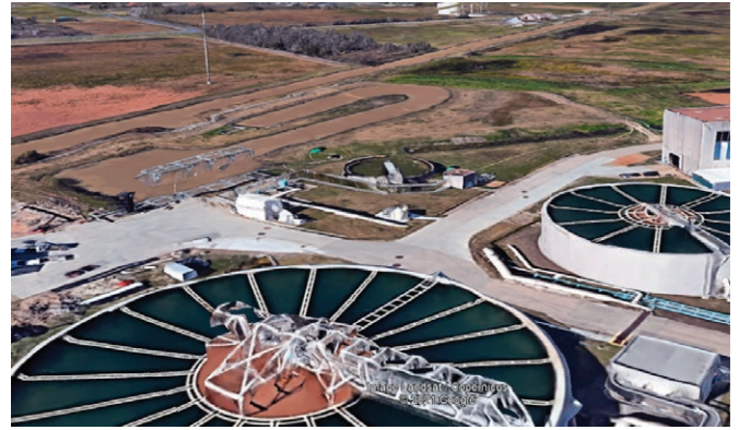
Treatment plant clarifiers with canal in background.
